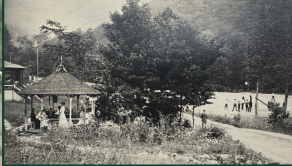
At left: Athletic Field, c1913. Above: Cooper Spring, Assembly Drive, and Ball Ground. Photo by Alice Margaret Dickinson.
